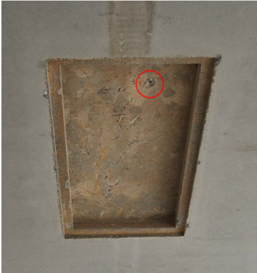
Hollow body after removal of the profile; Feed for speaker cables in red.
